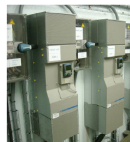
Figure 9 Variable Speed Drives in a pumping station
